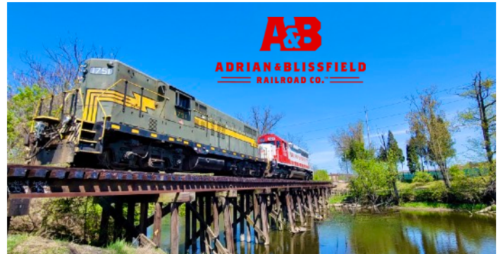
Adrian and Blissfield Railroad Bridge - Red Cedar River 2023
